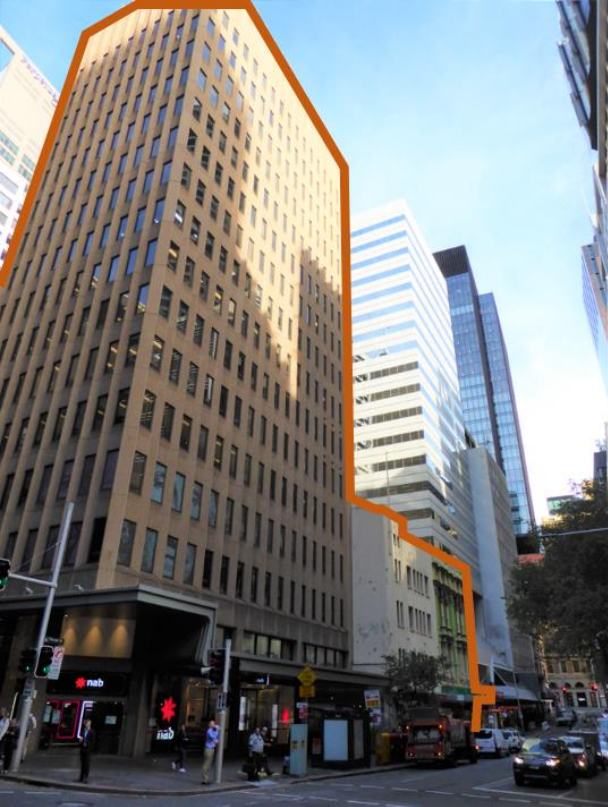
Figure 4: Subject site on the corner of Hunter and Pitt Streets, looking west along Hunter Street
